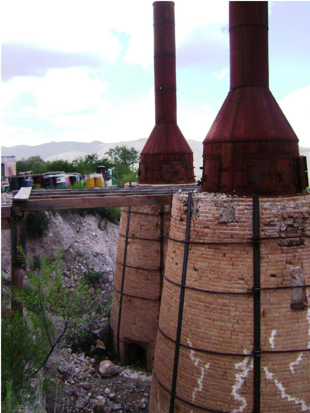
Figure 6-2 - Sierra Mojada Historical Lead Smelting Kilns - September 2010. These were removed in 2013.
